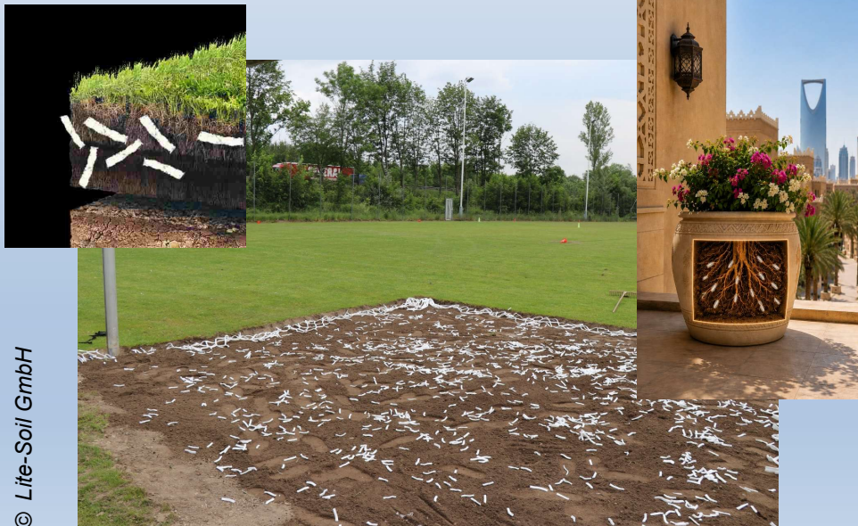
Subsurface textile water storage strips
