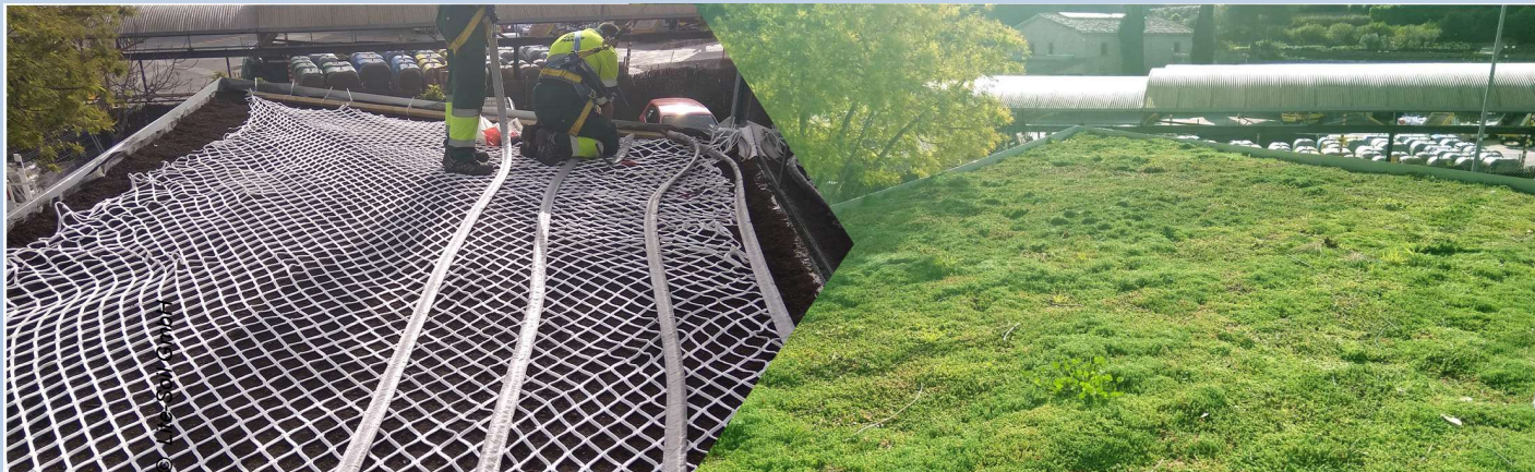
net-shaped textile with coated drip irrigation tubes (roof greening example) – system placed individually at root level
