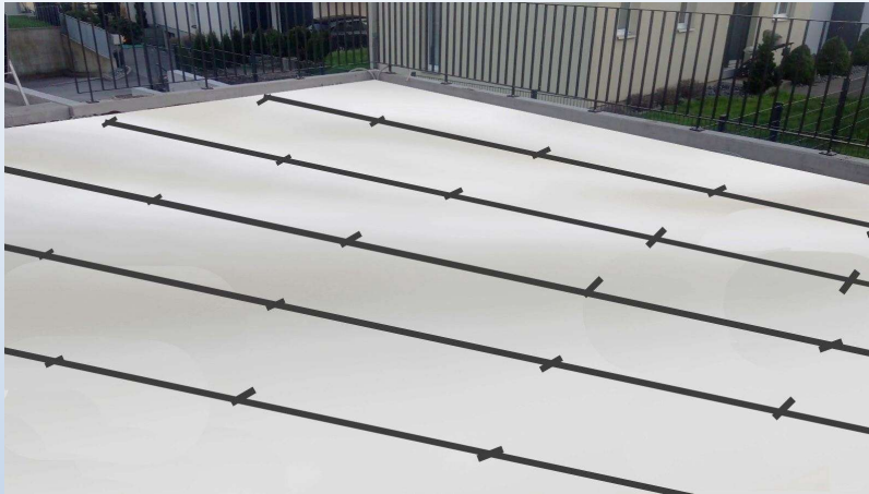
full-surface textile with non-coated drip irrigation tubes (roof greening example) – tubes placed on drainage layer
